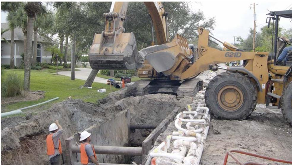
Figure 4. Gravity sewer main excavation.
