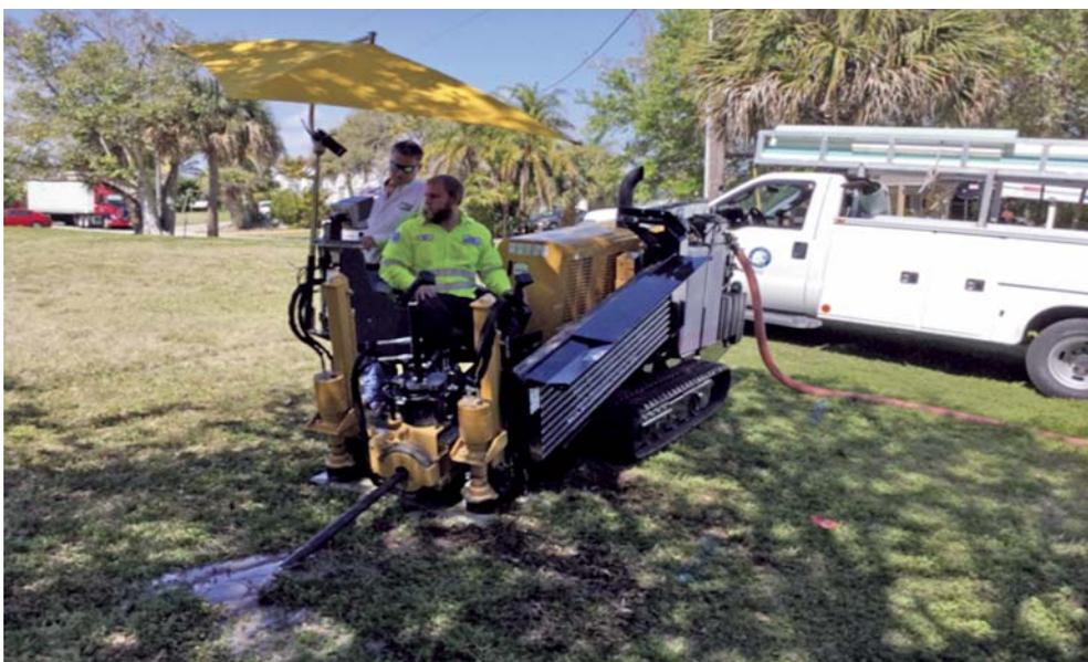
Figure 5. Directional drilling of 2-in. main.
